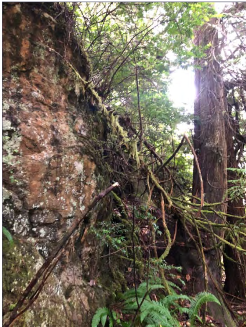
Figure 2.6.1 – Exposed Bedrock Above Access Trail (View looking East)
